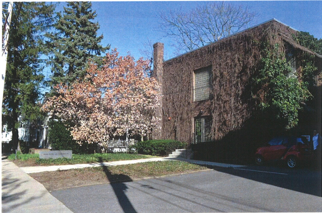
CURRENT VIEW FROM NORTH-EAST
